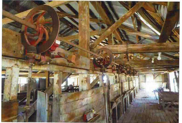
Dunlop Station shearing shed was the first to convert to mechanical shears
